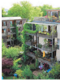
Dense, mixed tenure housing Vauban, Freiburg
